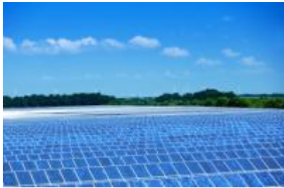
Figure 3: PV power plant
