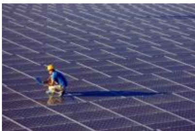
Figure 1: Large PV covered roof in Germany
